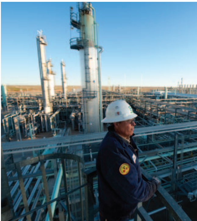
Seminole Gas Processing Plant, Texas
